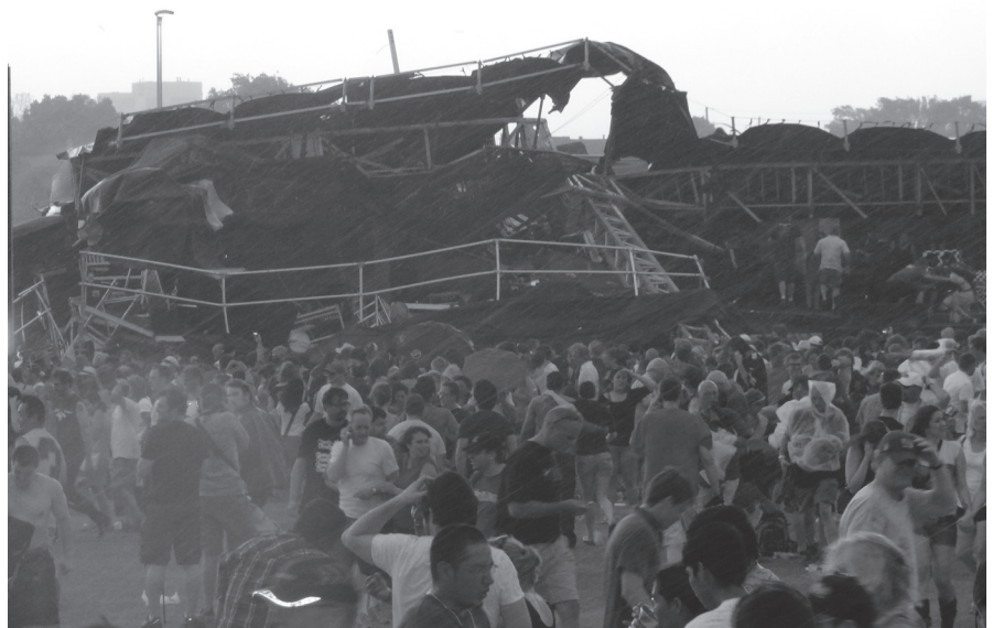
Collapsed stage at Ottawa Bluesfest. Photo: Sandra Luty
